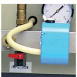
Immediately open the discharge valve slowly and the fuel will run out, purging the air from the discharge pipe, which will flow out through the open vent cock. The discharge pipe now being full of fuel and having no air makes it possible to start the appliance.
