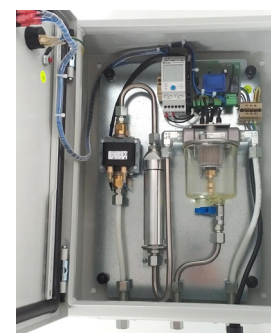
MicroSAFA in IP66 cabinet, with adjustable timerswitch
